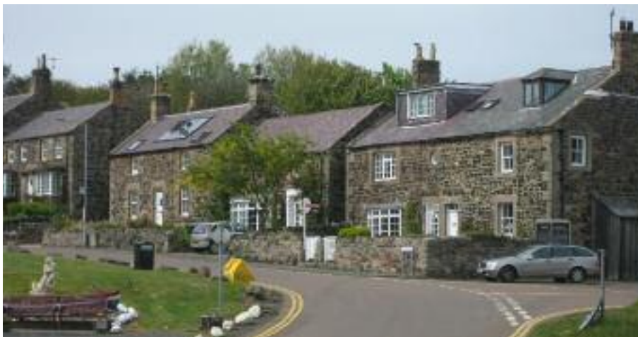
Cottages at Craster are built mainly of locally quarried undressed 'whinstone' rubble from the Whin Sill. Quoins, lintels and window casings are mainly of Carboniferous sandstone of unknown provenance. The roofs are of Welsh slate.
