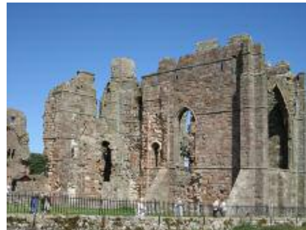
Lindisfarne Priory is built mainly of Carboniferous sandstone, perhaps obtained from the Cheswick area. Locally sourced stone, including Whin Sill dolerite, may be seen in the exposed rubble cores of many of the walls.
