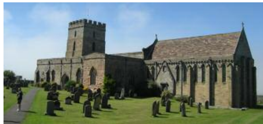
St Aidan's Church, Bamburgh is built largely of locally worked Carboniferous sandstone, with Carboniferous sandstone slabs roof tiles (of unknown provenance). Memorials in churchyards such as this commonly employ a variety of rock types.
